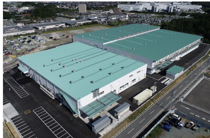
(Exterior view of Mie Mushroom Center)
